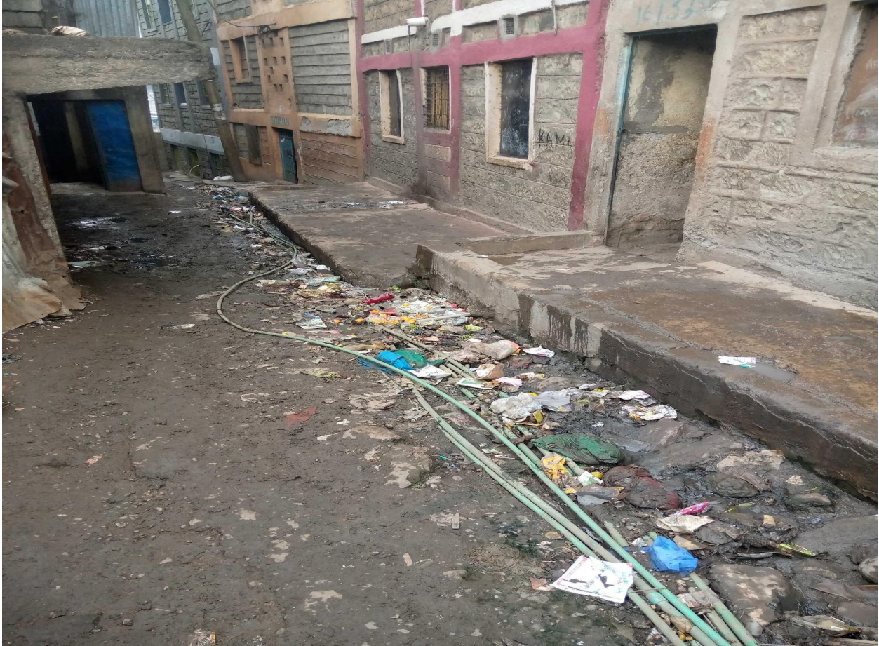
Plastic waste in a small trench outside a highrise residential building, a trench meant for draining waste water.
