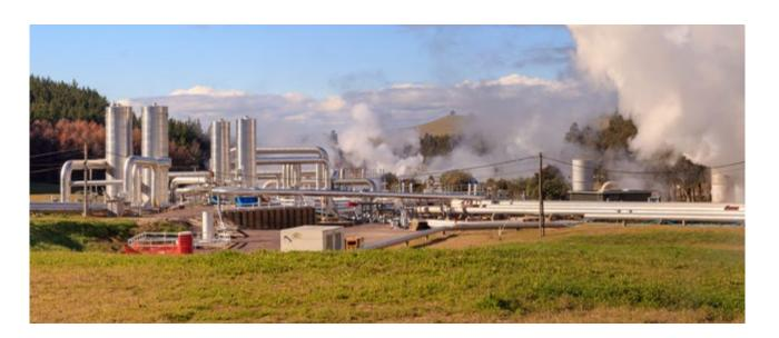
i Stand-alone closed-loop binary-cycle power plants can avoid significant venting of CO<sub>2</sub> and other pollutants from the geothermal fluid. Conventional open-loop power plants vent gases to the atmosphere.
